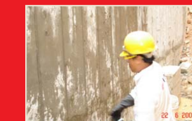
5. Prewatering before application
