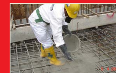
3. Sprinkling prior to casting
