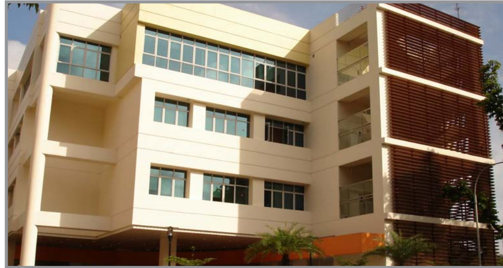
QUEENSTOWN POLYCLINIC - SINGAPORE
