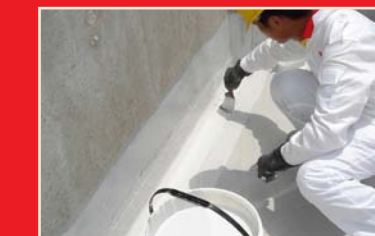
4. Coat Formak 629 over fibreglass
