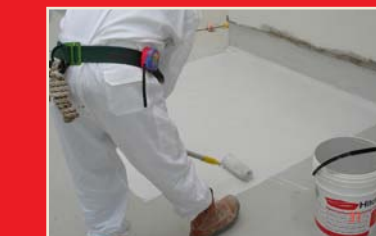
5. Application of 1st Formak Topcoat
