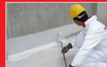
2. 1st Coat of Formak 629
