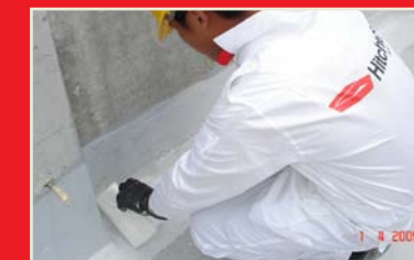
3. Unroll 100mm width fibreglass mat
