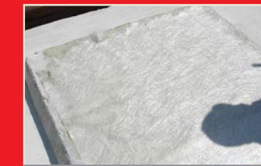
4. Unroll fiberglass over 1st bodycoat
