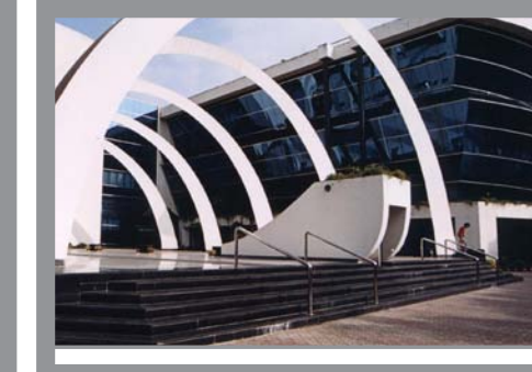
◀ Tata Internet Building - Mumbai India
